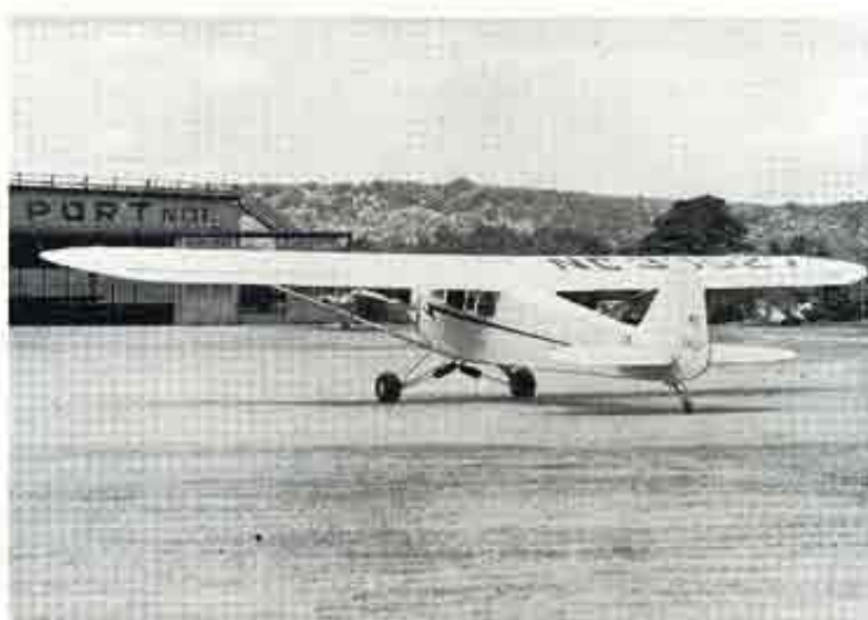
52. When ship has slowed down to approximately 15 m.p.h., turn off runway and S-taxi slowly toward the hangar, watching out for other ships.
